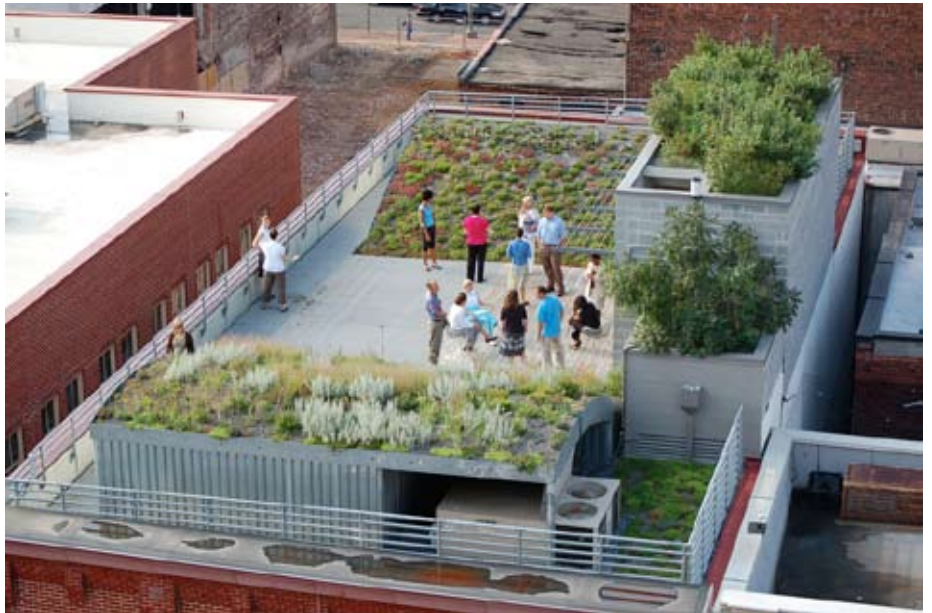
The green roof on the headquarters of the American Society of Landscape Architects in Washington, D.C. was completed in 2006 and is a showpiece for aesthetic design and environmental benefits. American Hydrotech, Inc. supplied the Garden Roof® Assembly components for the green roof.
