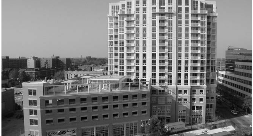
The Church Street Station Condominiums Green Roof Project in Chicago, IL.
