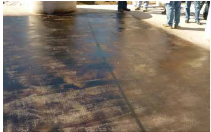
Surface conditioner applied
