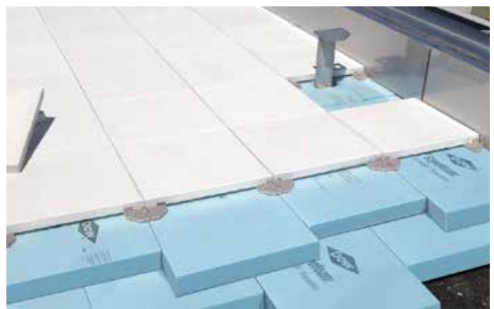
Concrete pavers installed
