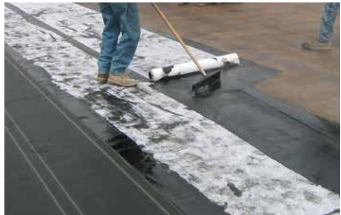
Membrane application in field of deck
